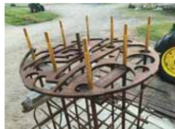
Subframe showing rebar, vertical bolts and top steel plate.
