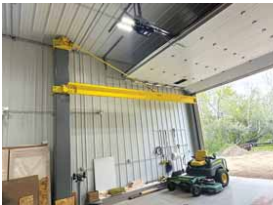
Gutschmidt recently built this shop hoist with subframe for his brother.
